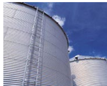
Fortunately, we have 'excess' oil storage
